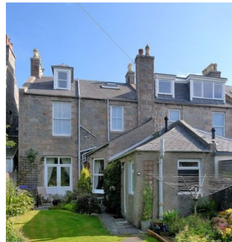
* Rear view of app site & ex. rear dormer @ 123 Blenheim Pl
