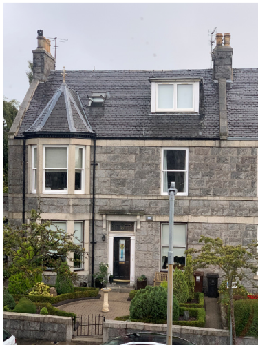
* Box dormer on Blenheim Pl front elevation
