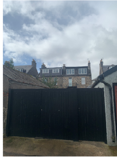
* Box dormer examples on Fountainhall Rd
